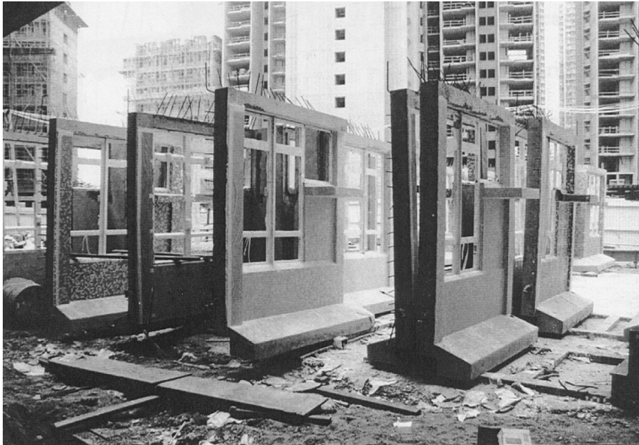
Precast concrete facades ready to be assembled and installed onto the floor slab
