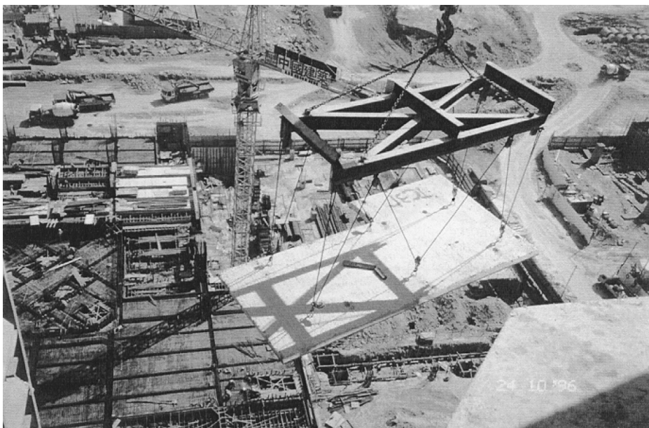
Precast concrete slab being hoisted into position
